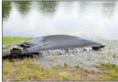
Plate 4-6 Silt bag under inspection
