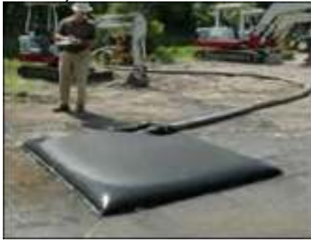
Plate 4-5 Silt bag with water being pumped through
