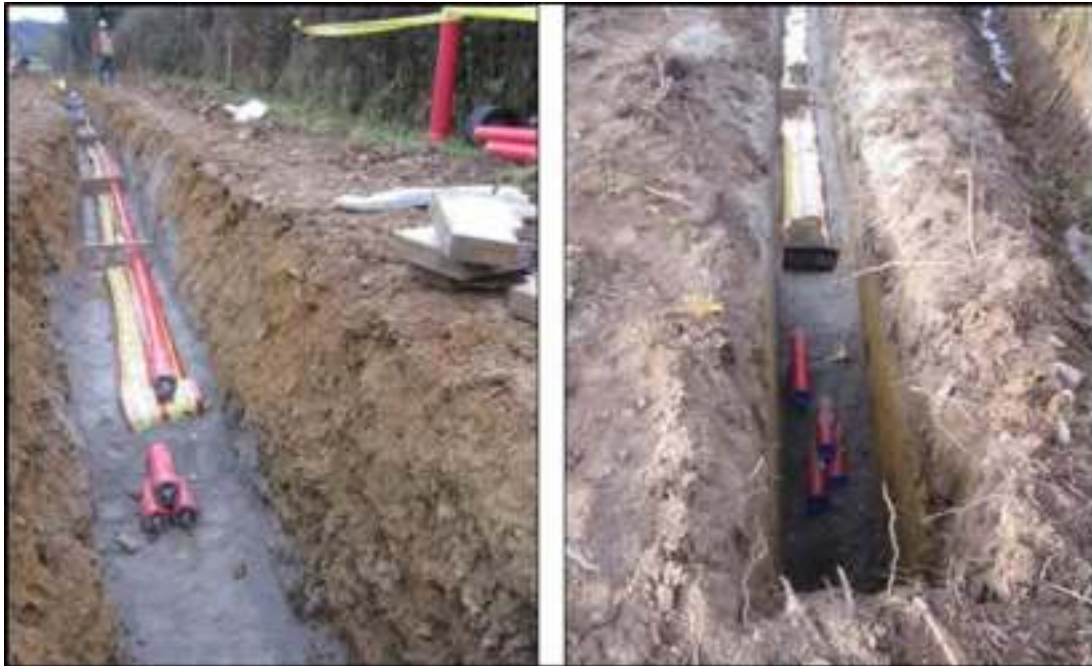
Plate 4-7 Standard Cable Trench View
